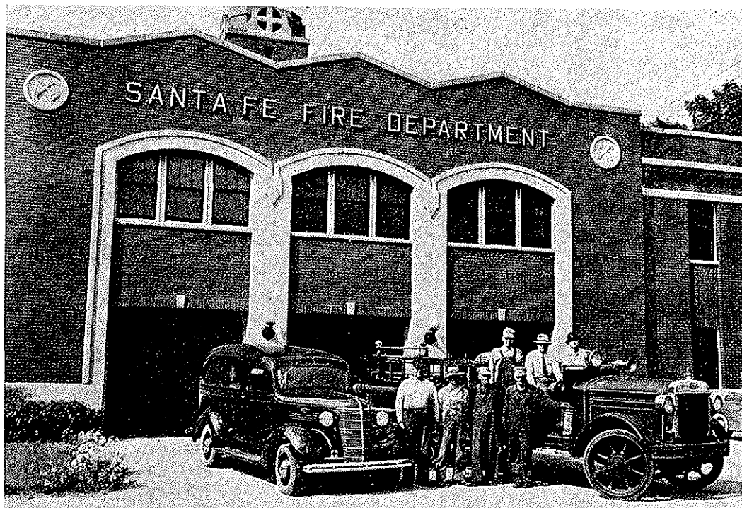
The Santa Fe's power plant and electrical equipment supervisor and inspector is responsible, among many other things, for the general inspection of fire prevention and fire fighting equipment at roundhouses, shops and terminals. Above is shown the Santa Fe fire house and crew of the Topeka shops.
