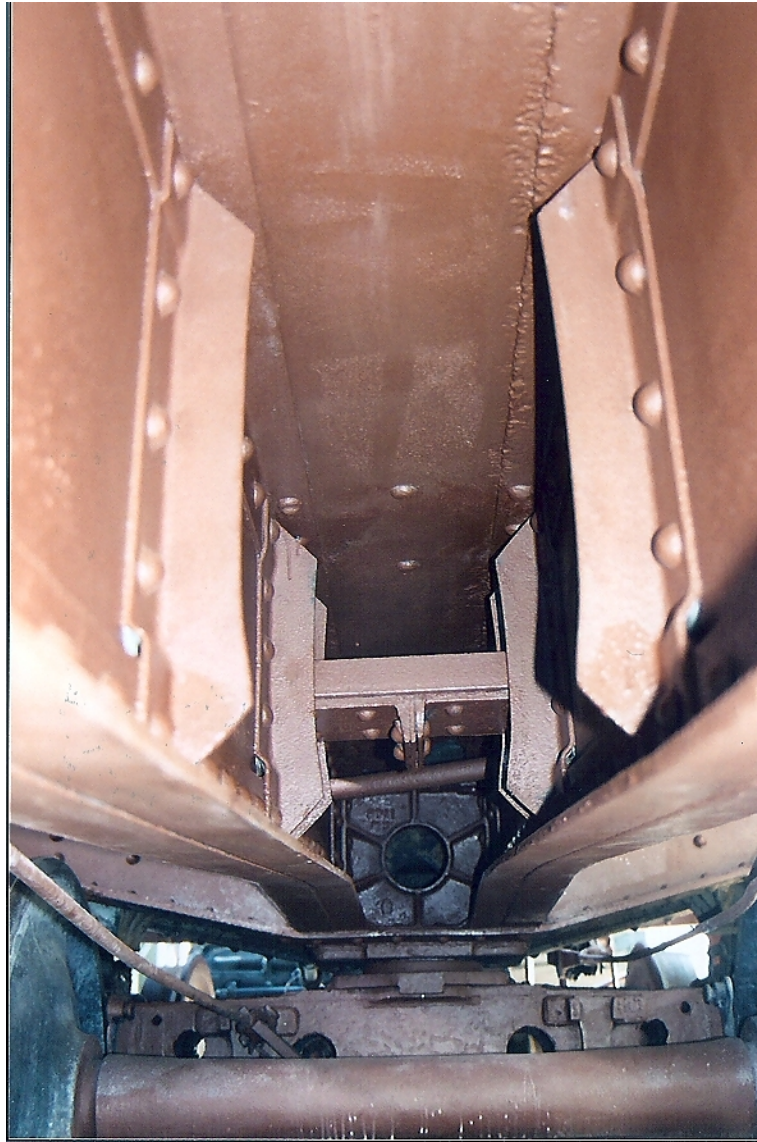
Figure 11. B end centersill after cleaning and priming.
