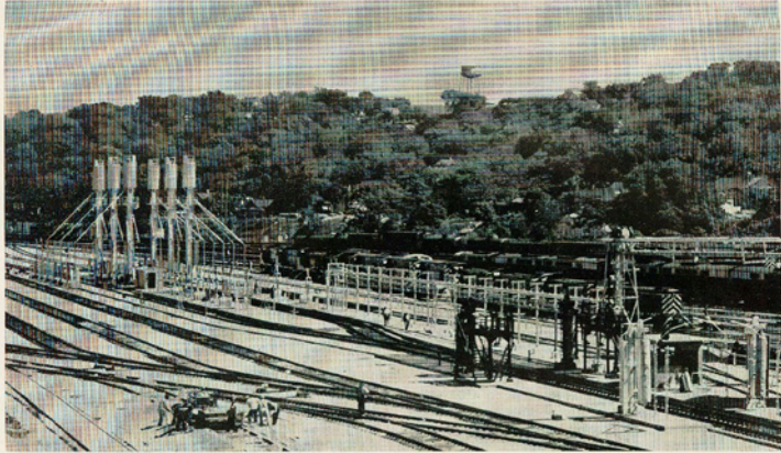
SERVICING OPERATIONS are divided into three principal groups: Sanding; fueling, watering and lubrication; and washing. Engines enter at sanding station (left) and
