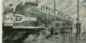
1 SANDING is performed at first stop from elevated steel platforms with retractable sections which permit attendants to stand close to engines.
